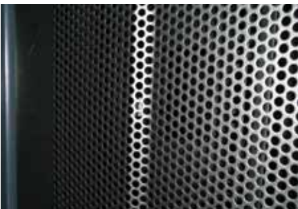
Perforated doors enhance ventilation
