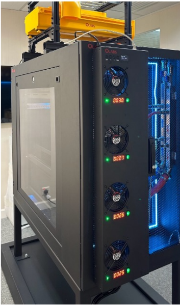
Master Smart Fan Unit (OIF-R4M-1) Rear door 4 fans – extract airflow
