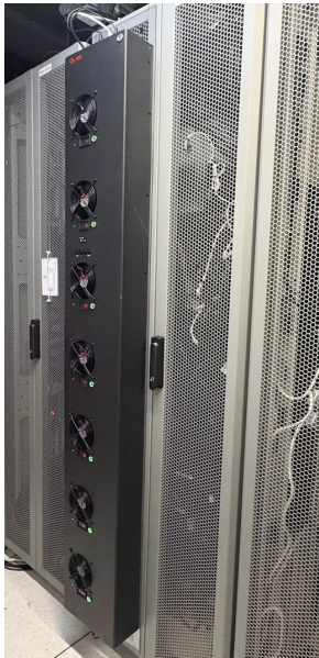
Master Smart Fan Unit (OIF-R7M-1) Rear door 7 fans – extract airflow
